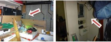
Several breaker(s) turned off. Unable to determine reason. Oversized circuit breakers and doubled up circuits noted.
