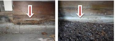
This area is susceptible to deterioration and possible wood destroying insect infestation. Concealed issues may exist. We suggest removing earth from base of wood and repair of any deterioration as needed by a licensed contractor. Boards weathered/deteriorated at right side.
