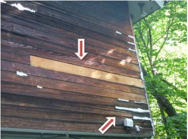
Areas patched. Unable to determine if, or to what degree, water has penetrated behind this siding. Concealed issues may exist. Suggest confirming/repair as needed.
