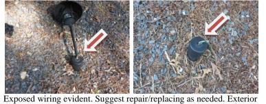
outlets do not appear GFCI protected. Suggest installing approved ground fault protection for safety. We check a representative number of
