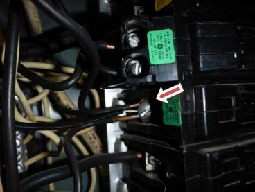
This condition can allow excessive current to be carried by the conductor causing overheated wiring and possible fire. Several panels in this home were manufactured by Federal Pacific.
