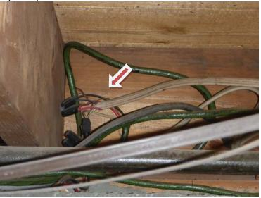
Light(s) appear permanently wired with lamp cord. Suggest repair as needed.
