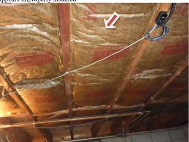
Suggest repositioning against heated space above and insulating where not present.
