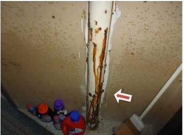
Portions of these columns appear to have been replaced with temporary style jack columns.
