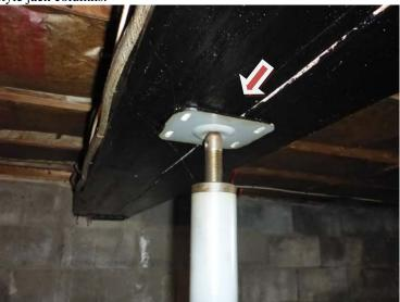
Suggest installing approved, permanent type columns with proper footings below this beam.
