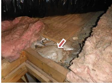
Suggest removing all vapor barrier material other than layer against heated space below and insulating over pull down stairs. Soffit and ridge vents.
