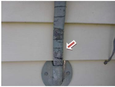
Meter box loose. Suggest repair/replacing as needed by a licensed electrician. Exterior outlets are not ground fault circuit interrupter (GFCI) protected. Suggest installing approved ground fault protection for safety. We check a representative number of exterior lights. If concerned, we suggest confirming operation of all exterior electrical fixtures.
