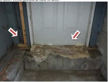
Water penetration evident sometime in the past. Floor drain present in this area. Unable to determine effectiveness or where drain terminates. Suggest repair as needed.
