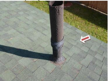
Leakage possible sometime in the past. Unable to determine if active. Suggest monitoring/repair as needed.
