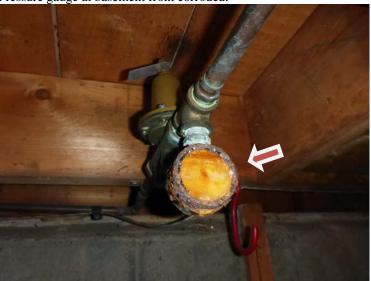
Suggest replacing. Portions of basement piping not well supported. Unable to view supply piping in basement where walls/ceilings are finished.
