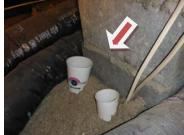
Underside of roof sheathing sealed with what appears to be roof cement.
