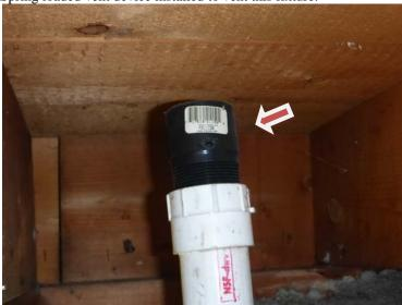
These devices are generally not permitted as they can fail allowing waste gas entry into the area. Suggest installing an approved air admittance valve or extending this vent piping to the exterior by a licensed plumber.
