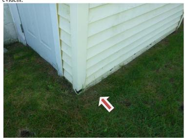
Unable to determine if deterioration has occurred behind vinyl. Suggest confirming, removing earth from base of siding and managing water away from this area to prevent water penetration and deterioration.
