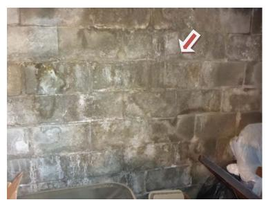
This indicates moisture and/or water penetration sometime in the past. Unable to view foundation where walls are finished or blocked by stored items.
