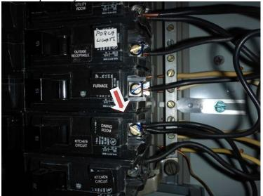
Generally, this condition is not allowed or approved as the termination lugs are not designed for multiple wires being attached and should be independently fused for better protection. Suggest confirming adequacy/repair as needed by a licensed electrician.
