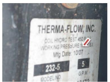
Client should anticipate replacement. We do not warrant the amount of hot water tankless coils will provide. With age, these coils can corrode and become restricted.
